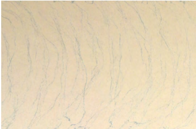
COVERAGE TOO LIGHT
